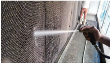
CoolPads can be cleaned easily with a high-pressure cleaner.
